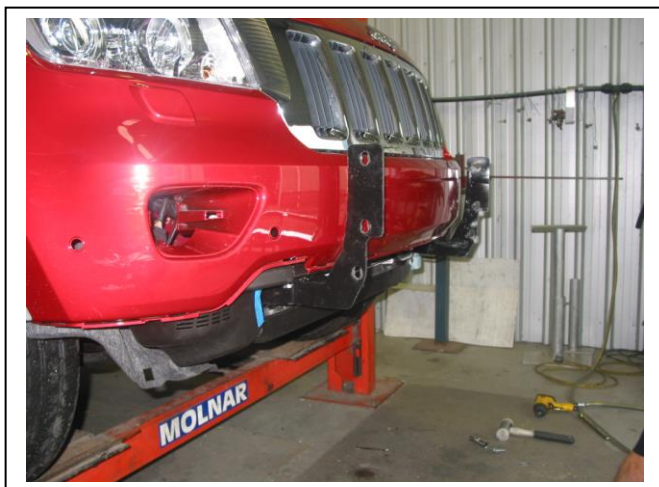
Figure 5: ECB steel mounting brackets fitted.
